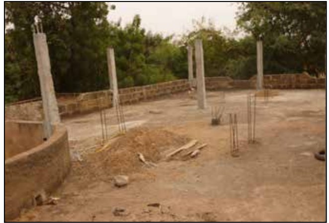
Covered shelter under construction
